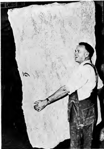
Fig. 8. Rough-surfaced stone slab, spray-cast from mixture of chopped glass fibers and plaster slurry by Paralite process.
